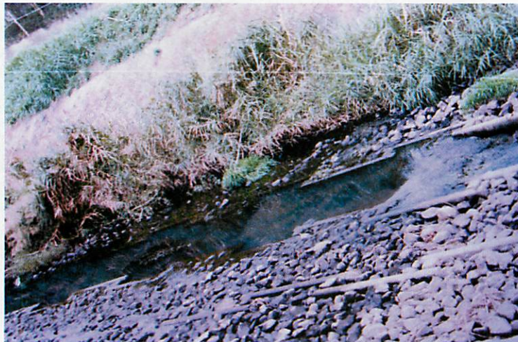
Fig. 6 Stones fixed with wooden frames
